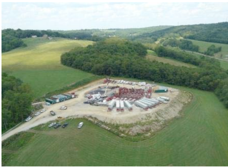
Figure 12: Well Site during Hydrofracturing
